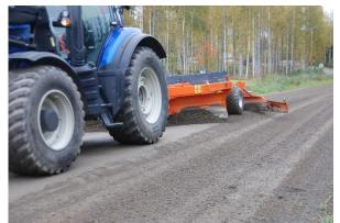
Picture 3. There is enough material on the road, which makes leveling possible. Leveling eats the tires. Petri has two sets of tires. Better vane tires with spikes are for road maintenance in the winter time, also for the operation in conurbations. Worn out vane tires still usable for summer time jobs.
