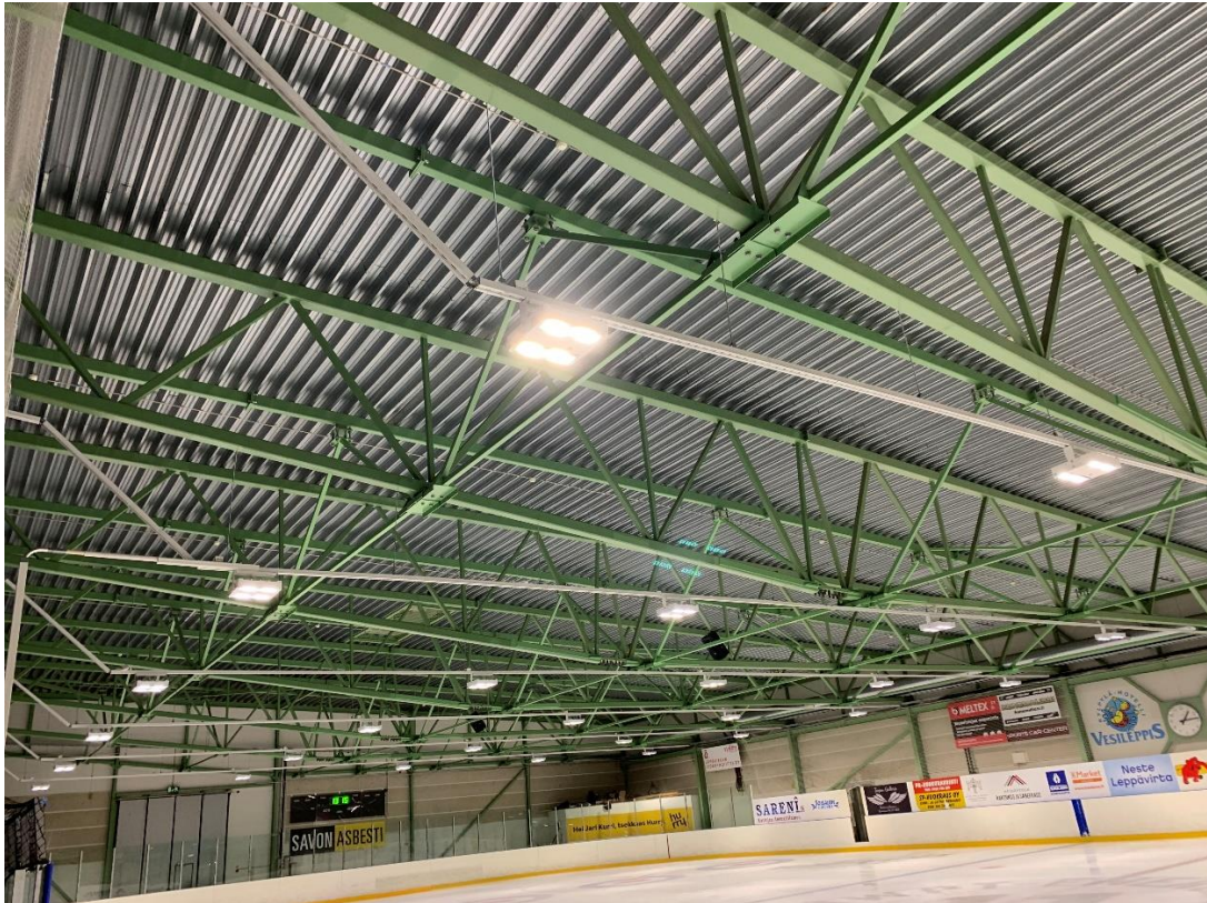
Picture 4. Leppävirta Ice Hockey Hall, the current wall and ceiling support structure with the reinforced structure.
