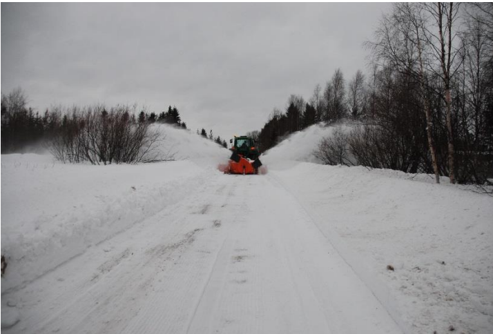
Picture 6. The snow cannot be thrown on either side in many places. If the snow can be thrown to the other side, operation is easier. The blowed snow does not break the surrounding structures, so the snow can be thrown into the trees.
